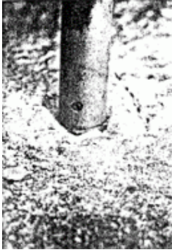
Drill until the anchor is 2 mm to 3 mm below the surface
