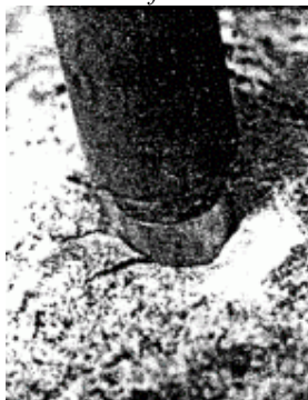
Sideways pressure can cause the rock to crack
